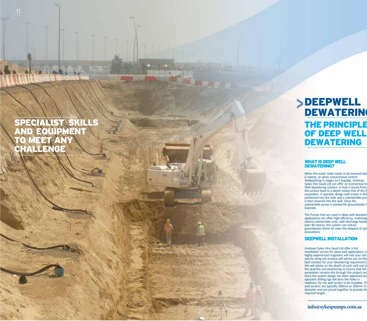
The wells are often surrounded with additional filter media to aid drainage and prevent fines from entering the system. Once the well has been flushed it is ready to have the borehole
